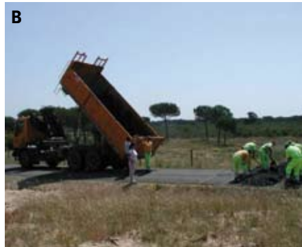
FIGURE 2. (A). FAUNA UNDERPASS PLACED IN A ROAD OF DOÑANA AREA. (B). CONSTRUCTION OF SPEED BUMPS IN A ROAD OF DOÑANA AREA.
